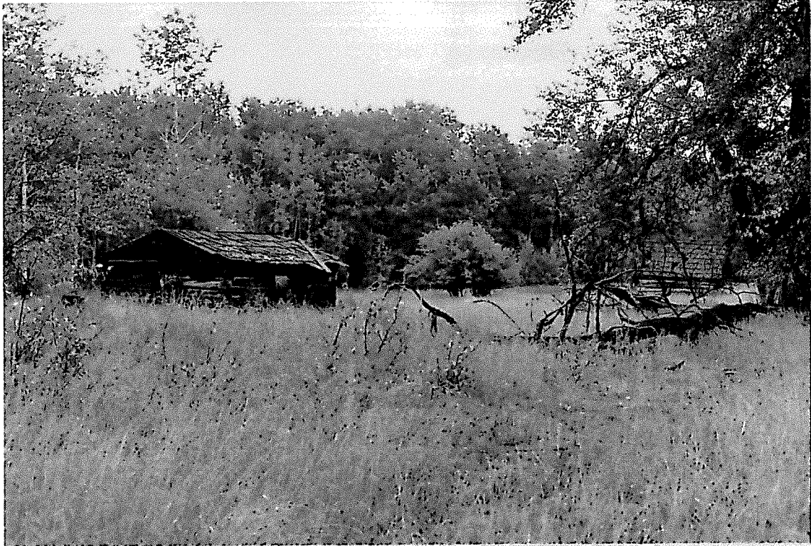
Figure 19. D1Rd 6, looking north at log house (HF 2) and barn (HF 3).
