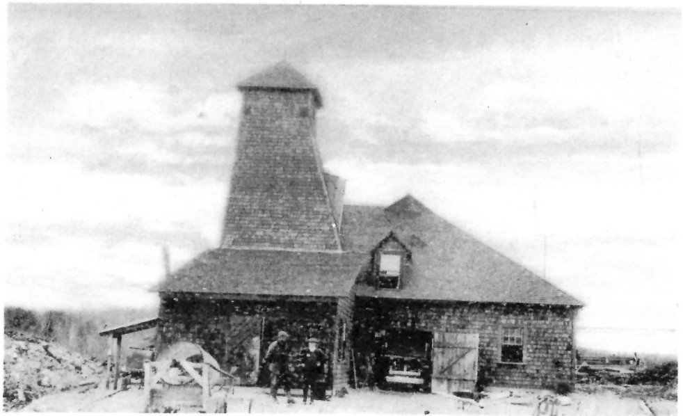
A. New shaft-house at Blackburn mine, range XI, lot 9, Templeton township, Que. The mica is rough-picked in the pit and dumped to the cobbing house in front of the hoist-tower, the clean, cobbled mica being shipped to the company's mica shop at Hull, Que.
