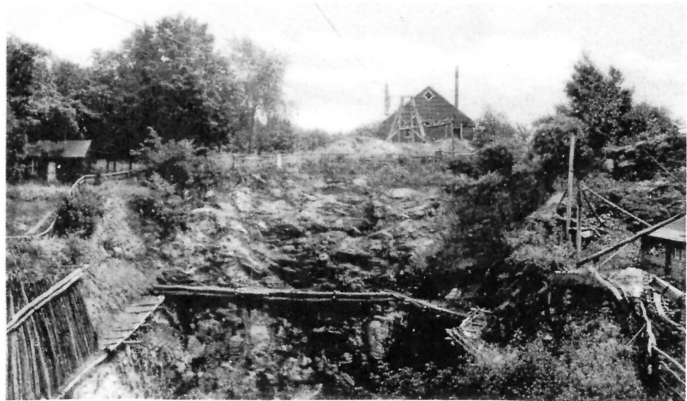
A. View of main pit, Lacey mine, concession VII, lot 11, Loughborough township, Ont. The strike of the mica leads is towards the hoist-house in the background, the principal vein (see Plate XV) passing approximately across the centre of the pit.
