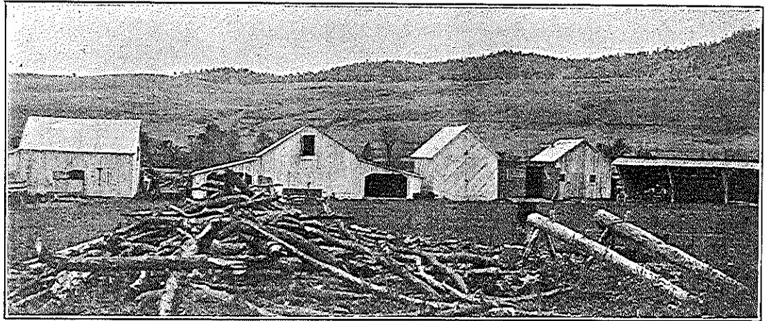
DOUGLAS LAKE RESERVE OUTBUILDINGS OF CHIEF JOHN CHILLIHEETZA
