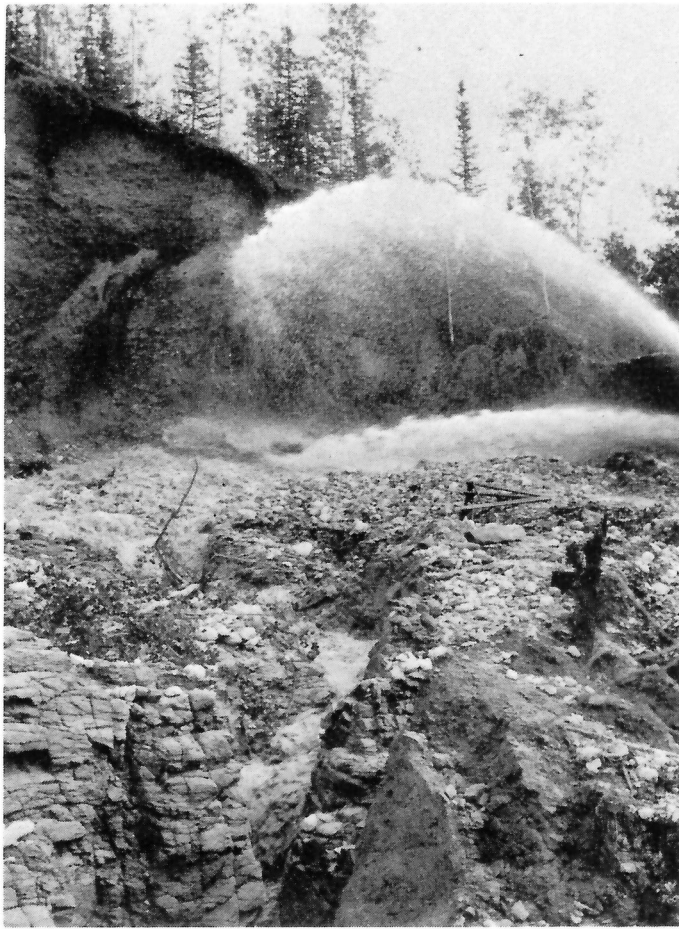
FIGURE 9 The start of hydraulic mining on Cripple Hill.
